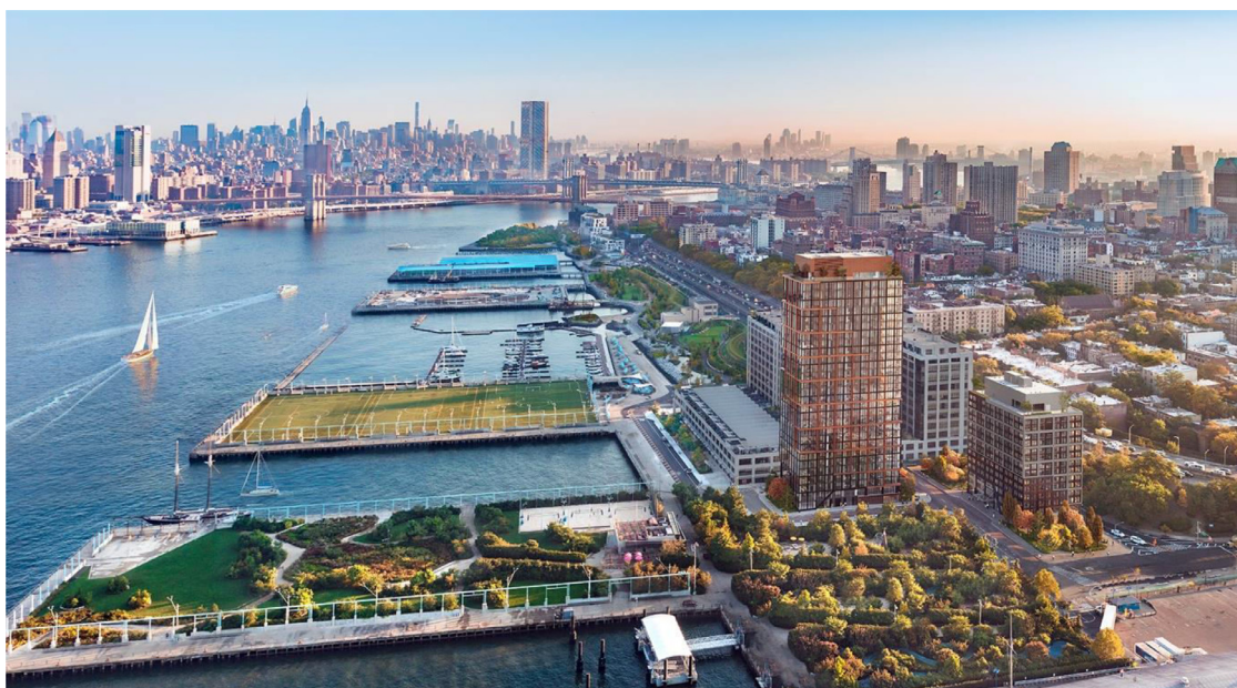
Figure 3. The Piers of Brooklyn Bridge Park (Pier 6 Ferry Terminal at the bottom of the image).
